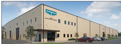
EVAPCO Key Building, Taneytown, Maryland
