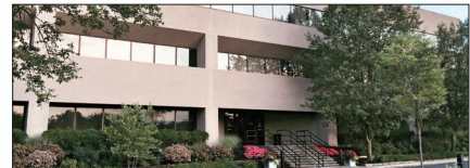
EVAPCO Dry Cooling, Bridgewater, New Jersey
