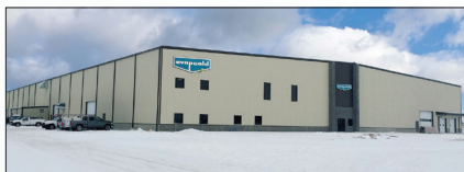
Evapcold Manufacturing, Greenup, Illinois
