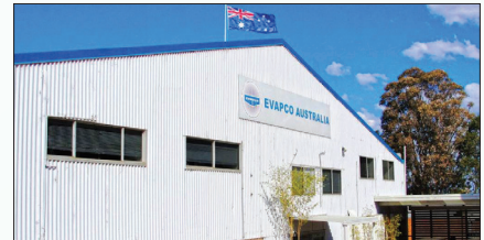
EVAPCO Australia (Pty.) Ltd., Riverstone, NSW Australia
