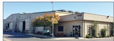
EVAPCO West, Madera, California
