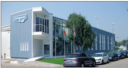
EVAPCO Europe, S.r.l., Milano, Italy
