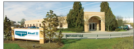
EVAPCO Alcoil, York, Pennsylvania
