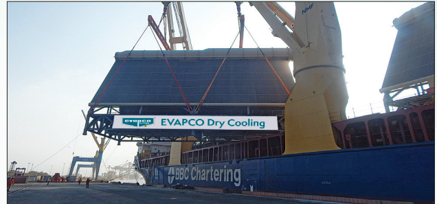
250-ton double fan module transportation
