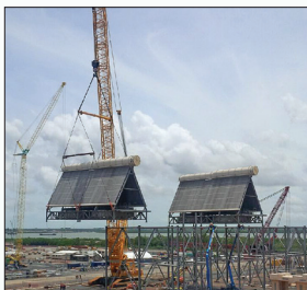
Modularization for efficient installations
