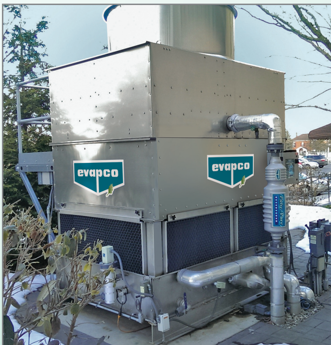
AT Cooling Tower with optional Pulse-Pure® non-chemical water treatment system
